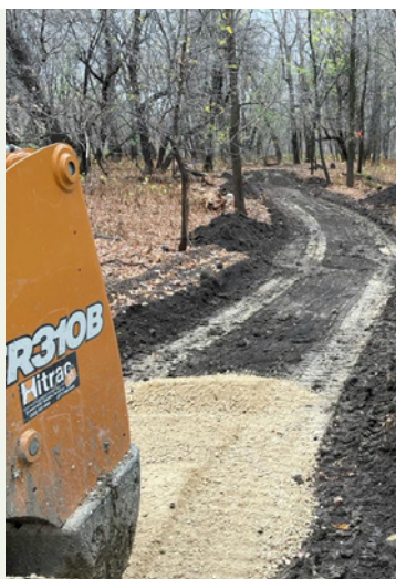
New Pathway Construction
