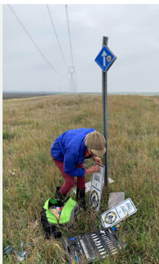
Signs on Floodway
